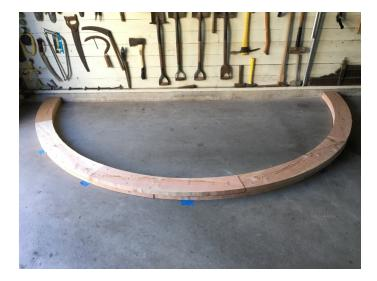
I did the same thing for the top half of the beam, leaving the two halves unscrewed. I screwed the vertical pieces to the top half in the shop. They will be screwed to the bottom half on site.
