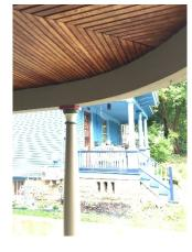
The architect was not willing to go along with my proposal as there are no charts to check on the strength for this unusual application. My gut told me that this method would create a very, very strong box beam, more than adequate for a span of about 4 feet. The old porch span was longer but the architect proposed five posts instead of the original three. After lot of e-mails and two meetings with the code dept. they agreed to allow my method of constructing the box beam.
