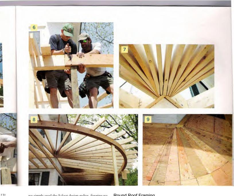
we simply used the 9-foot design radius, figuring we could persuade the beam ends into position with clamps.
