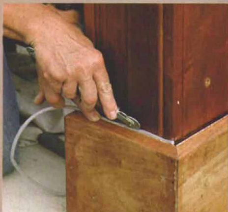
3. Backer rod allows caulk to flex.
