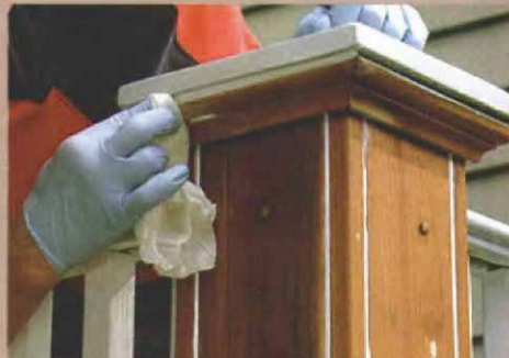
2. Mineral spirits remove excess caulk.
