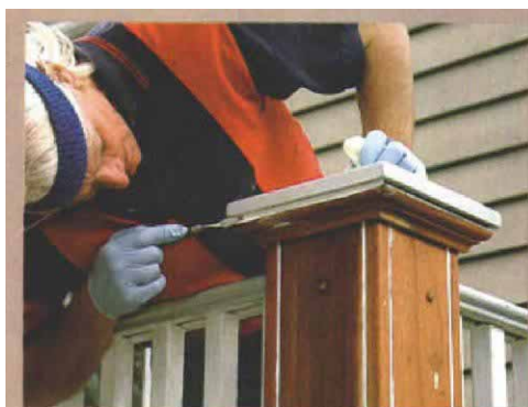
1. Palette knife tools visible joints.
