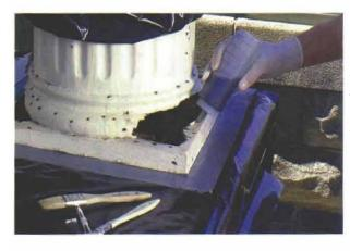
**Consolidant is injected into the repair.** Liquid epoxy, or consolidant, is squeezed into holes drilled around the repair. The consolidant saturates the soft wood, making it rock hard.
