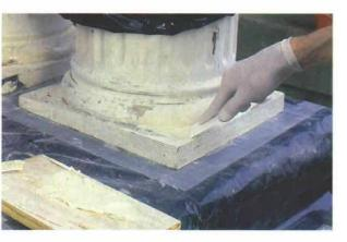
**Primer protects the epoxy.** As a final step before painting, a coat of primer is applied to seal the repair against moisture as well as against UV-radiation, which can damage some epoxies.
