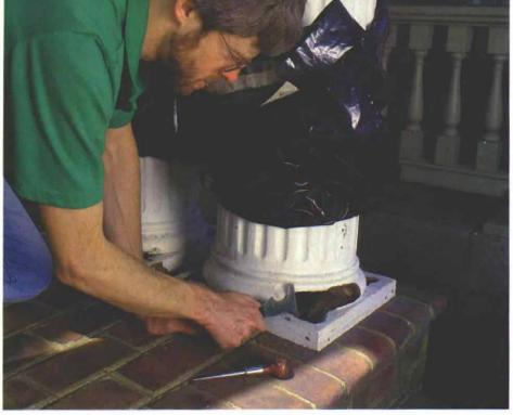
**Getting down to sound wood.** The first step is removing loose, crumbly wood. A five-in-one painters' tool and an awl are best for digging out any wood that is not still firmly attached.
