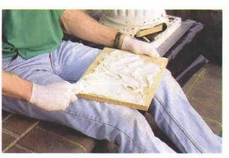
**Wood blocks save on epoxy.** To keep from using large quantities of expensive epoxy, blocks of wood are encapsulated in the epoxy to act as aggregate.
