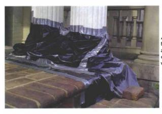
All dressed up. The same poly tent that is used to keep moisture away from the repair while it dries also protects the epoxy from weather while it cures.
